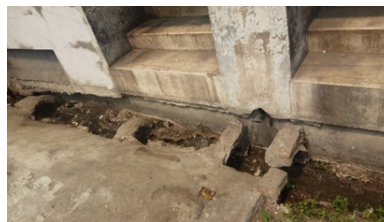
Figure 3 Open Drainage in 15 th segment
