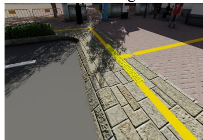
Figure 11 Design of Disabled Infrastructure Addition in the 1st Segment
