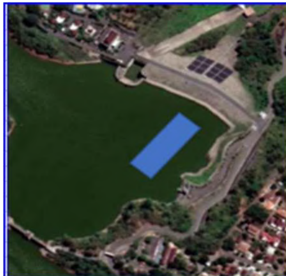
Figure 8. Location of Floating Solar Panel Source: Google Earth imaging 2021
