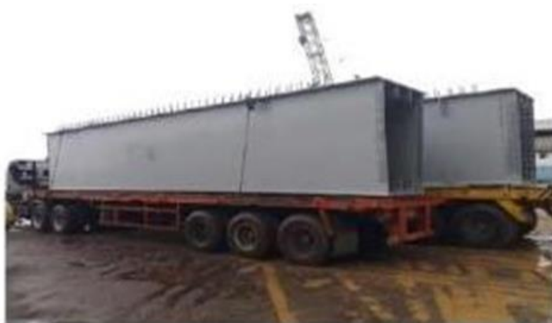
Figure 2. Delivery of segmental steel box girder
